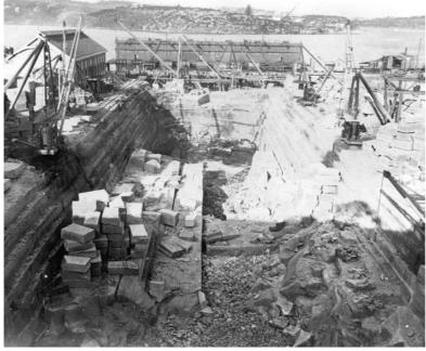
85,000 cubic metres of stone was cut out of the headland by the Morts Dock & Engineering Company creating a dry dock 188 metres long and 27 wide; at the time, the largest in Australia. It was used for repairs and fitting out of the sail and steamships that were the lifeline of the new nation. Once a ship tied up inside,
